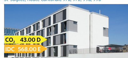
St-Sulpice, Route Cantonale 97a, 97b, 99a, 99b
